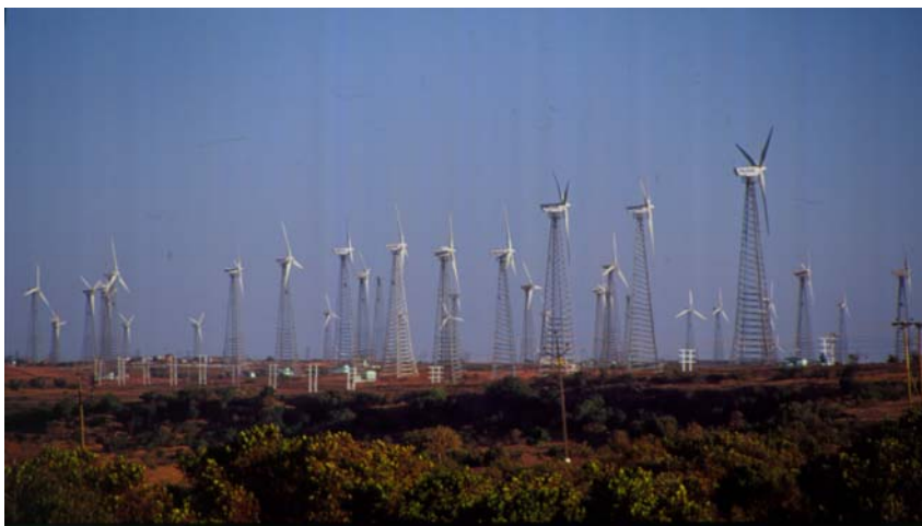
250 MW Capacity Wind Park at Satara
